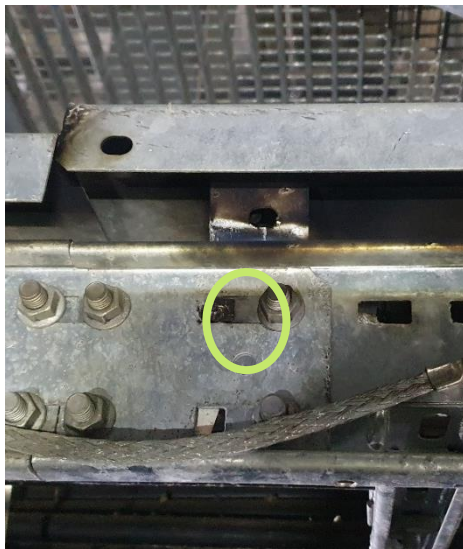
Hole drilled through tray
